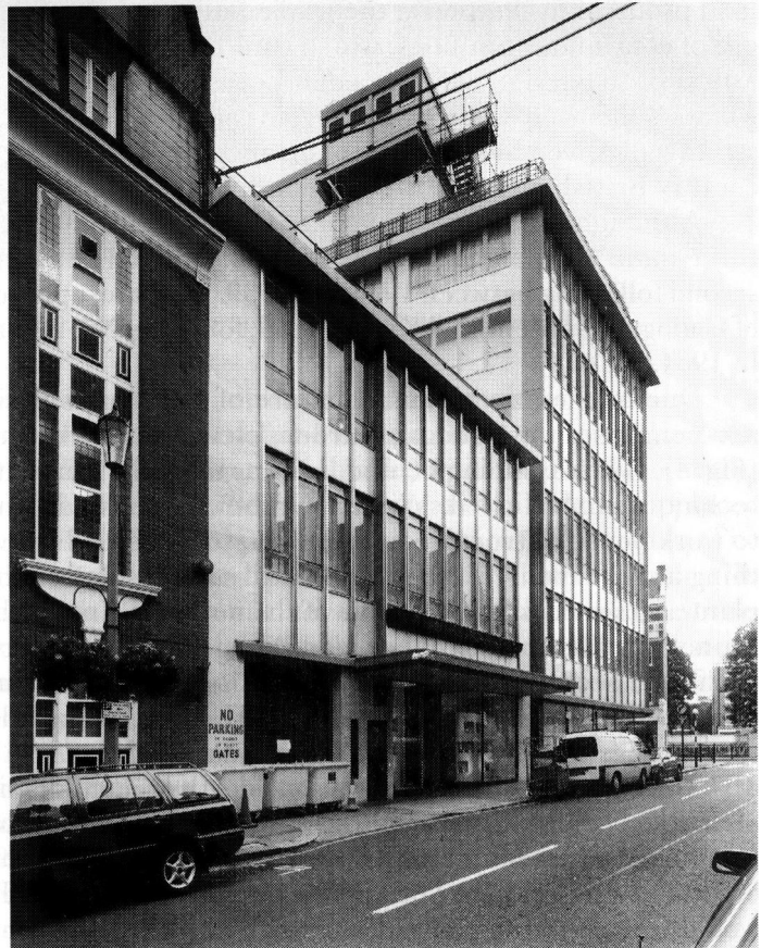
Fig 4 The Cadogan Gardens entrance (centre) showing the concrete mullions behind a metal facing and a cast- lead flower trough. Adjoining it (right) is the 1964 addition
